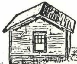
PASSENGER & FREIGHT DEPOT - ALLEN TOWN. - FROM PAUL H. STRINGHAM
