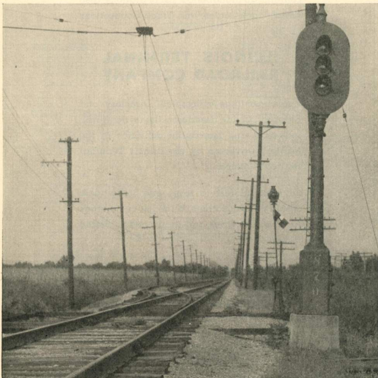
Right-of-way Scene on Illinois Terminal Showing Three-Position Automatic Color Light Signal
