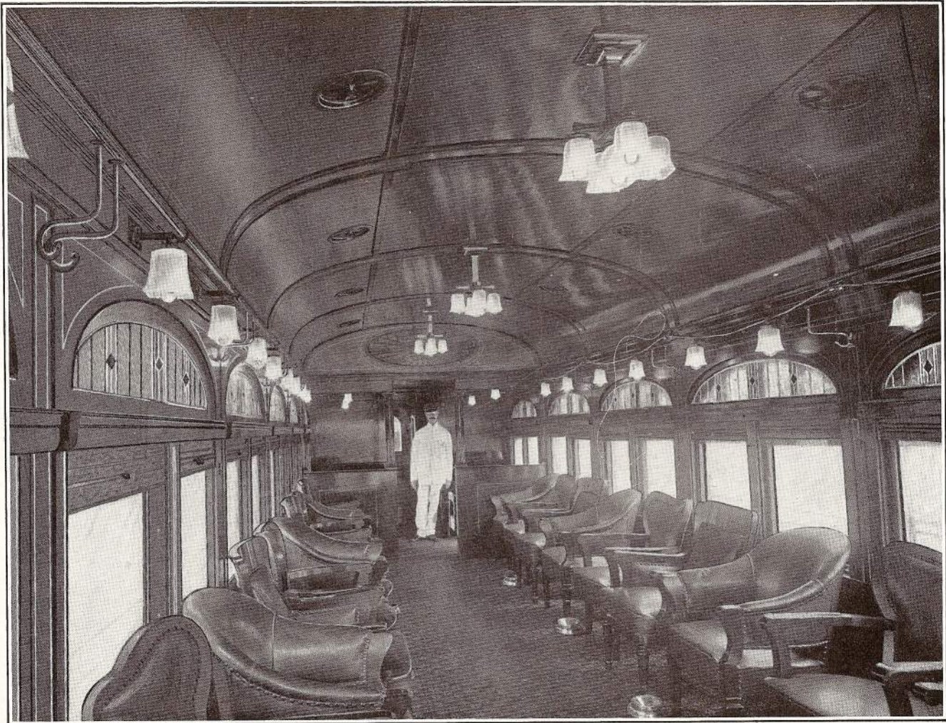
Interior Parlor Car
