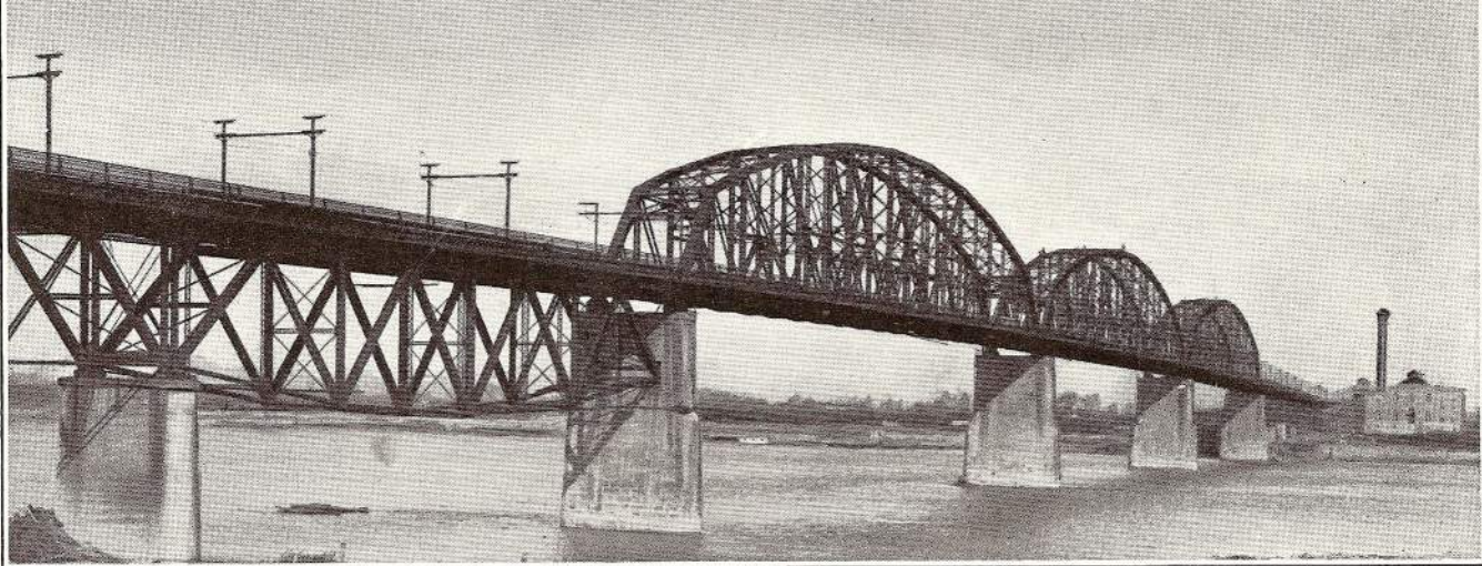
McKINLEY ELECTRIC BRIDGE
