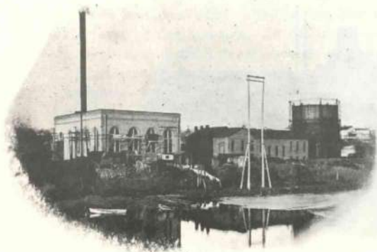
POWER HOUSE OF I. V. RY. CO.
