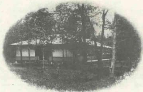
PUBLIC SHELTER AT DEER PARK.
