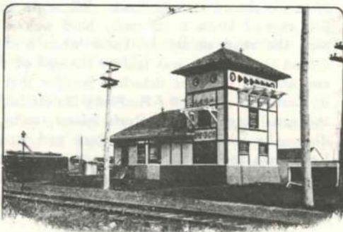
I. V. R. Y. CO. SUB-STATION.
