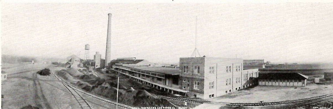
This is the plant of the Alton Box Board and Paper Company at Federal, Illinois. Although the smoke stack in this picture looks as though it were about to fall, it really isn't. The photographer probably was standing on one foot when he took this picture.
